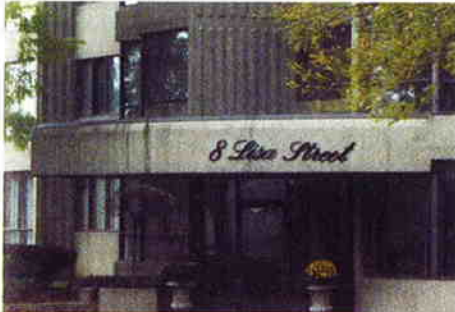
Cost-Effective Window Repairs
